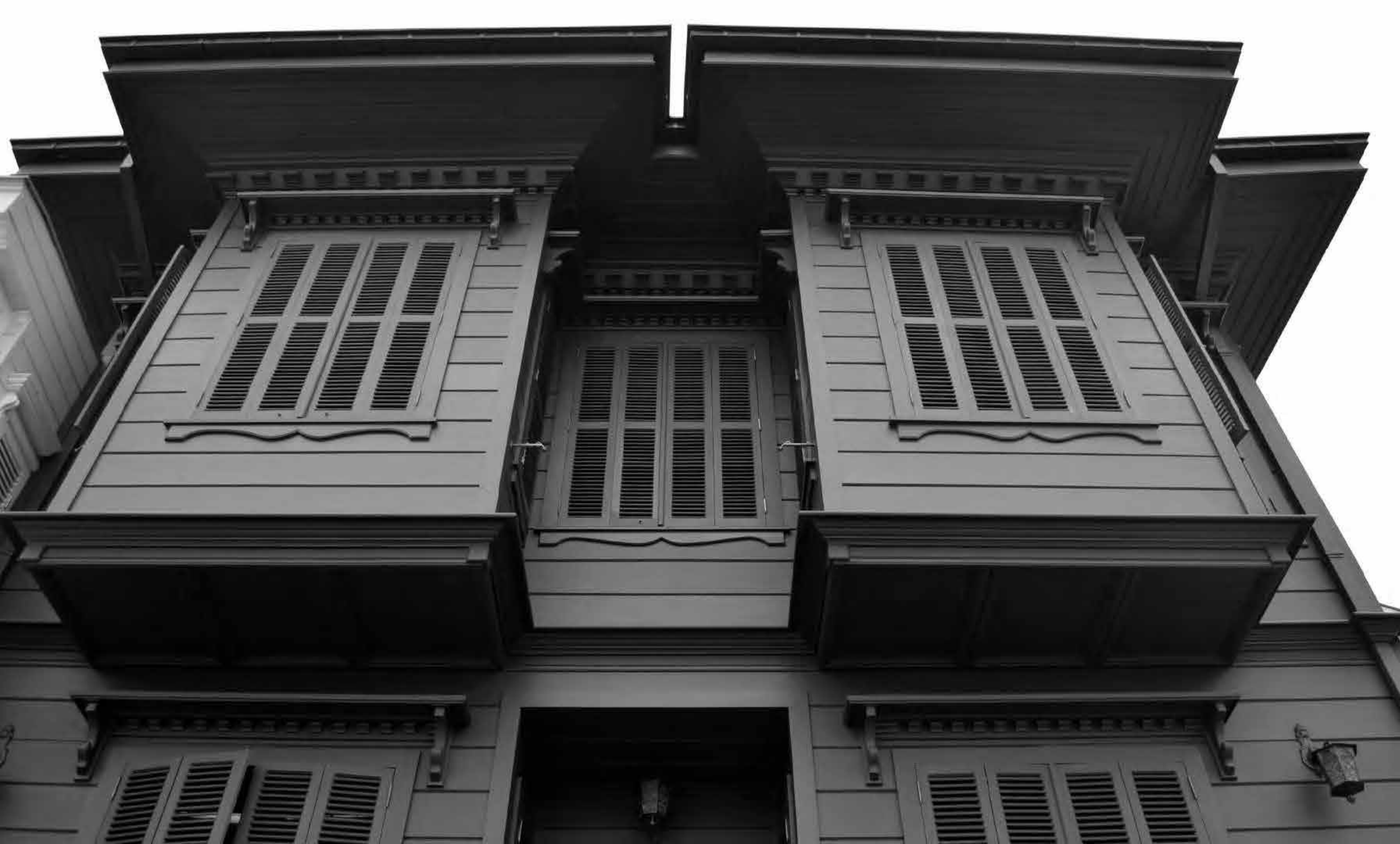
Niyazi Kaptan Waterfront Mansion Restoration Istanbul | Turkey 400 m 2
