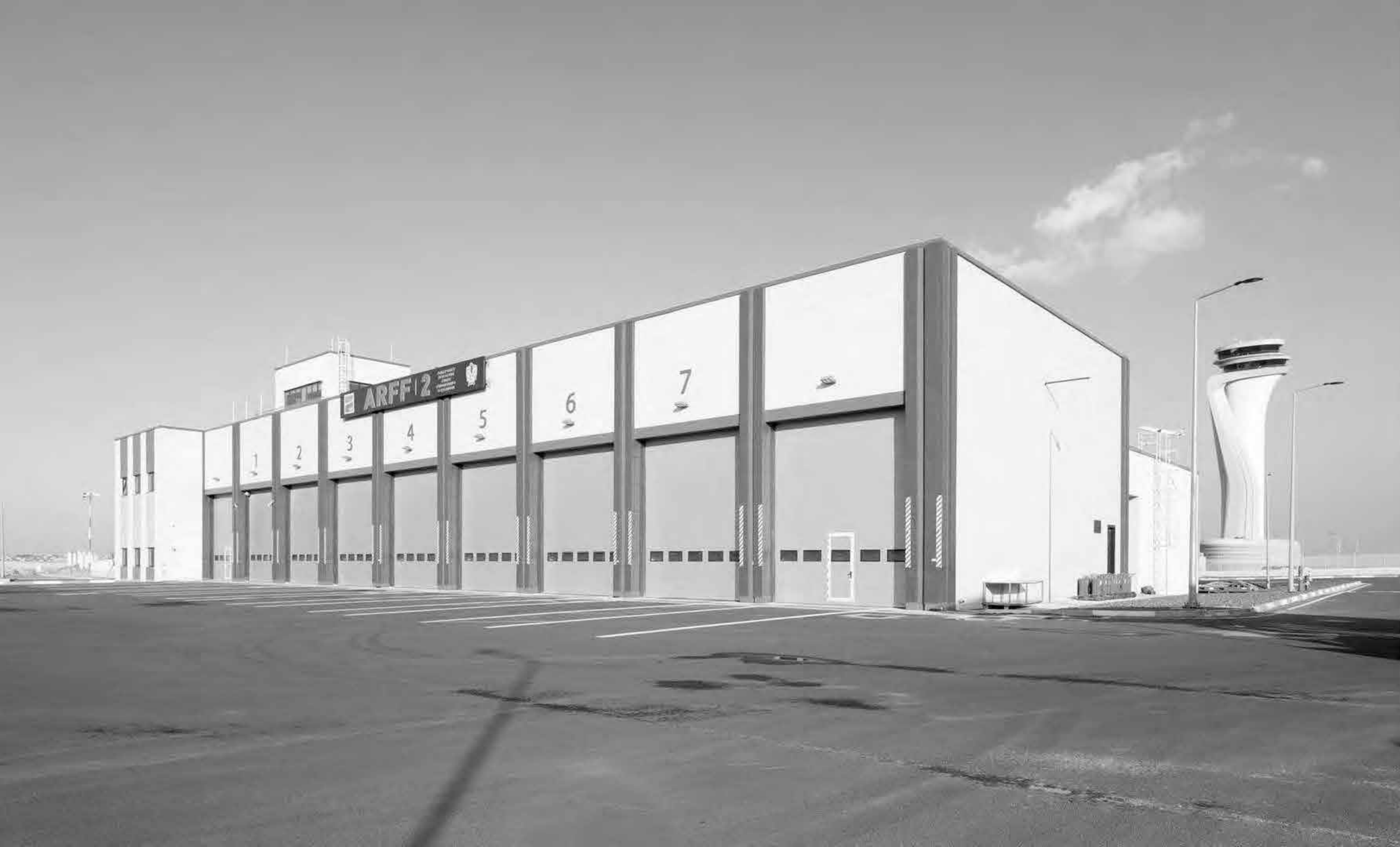
Istanbul New Airport Support Buildings Istanbul | Turkey 40.456 m 2
